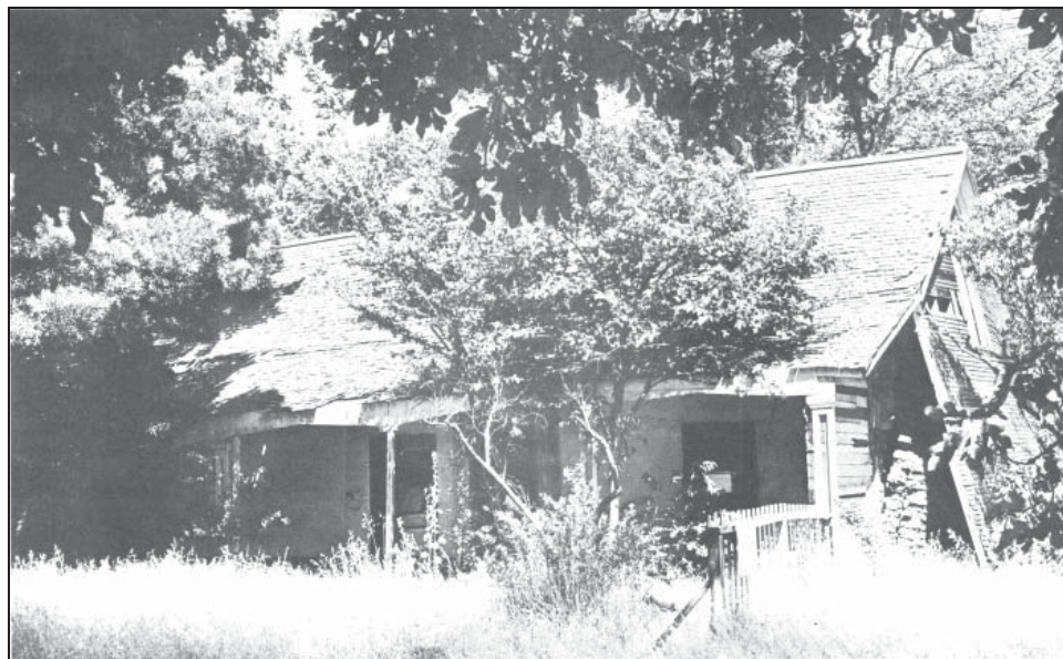
By the 1960s the Peña Adobe was in very bad condition when the Solano County Historical Society began restoration of the old structure.
