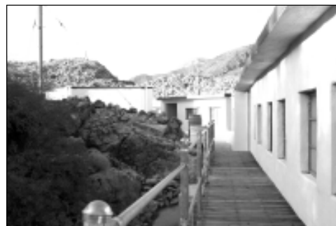
Boardwalk access to the 2nd floor bunk rooms ■
