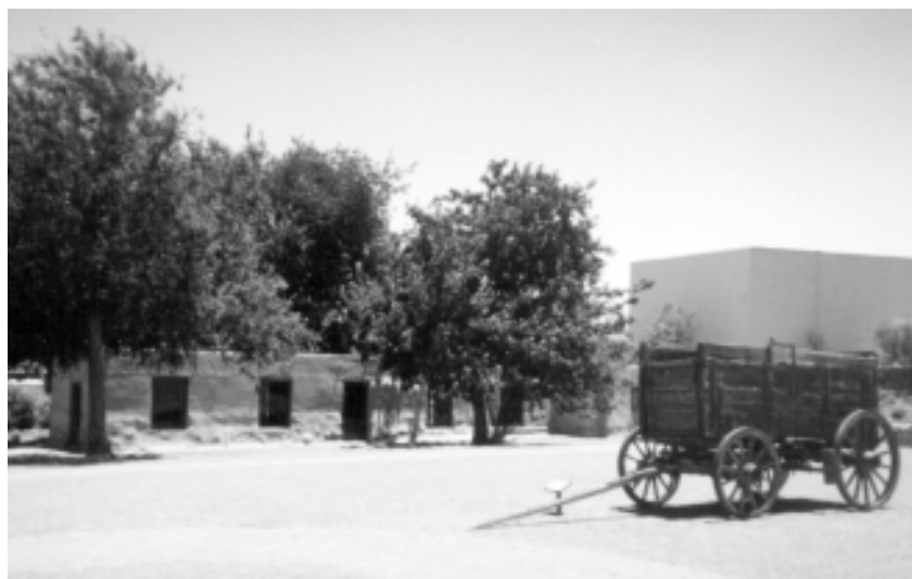
Las Vegas Fort under reconstruction. (Photo courtesy of Lou McCombs)
