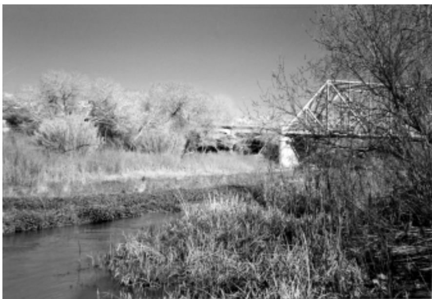
Route 66 bridge above Lane's ford.
